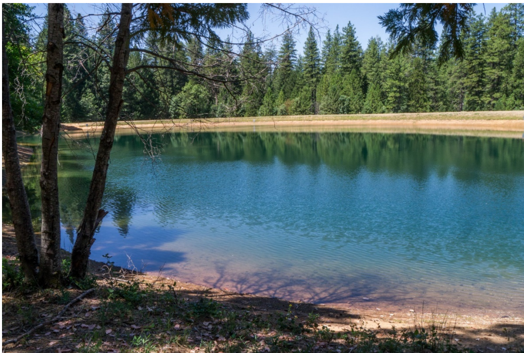
Nevada City operates a 55-acre-foot drinking water reservoir located in the middle of the BLM portion of the project area. Nevada City also operates a water treatment facility within the project area.
